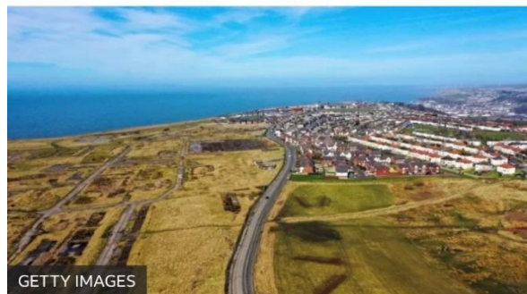
GETTY IMAGES The former Marchon chemical works on the outskirts of Whitehaven is the site of the proposed mine
